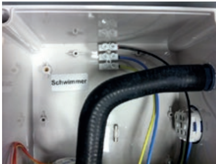
Figure 3: The hose inside the controller must not be twisted.
